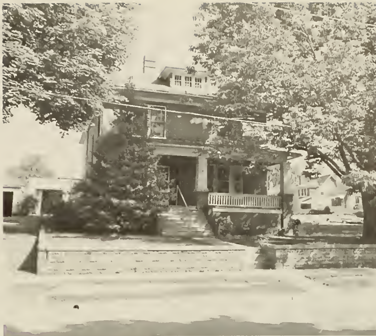
An exterior view of Wesley Foundation.
